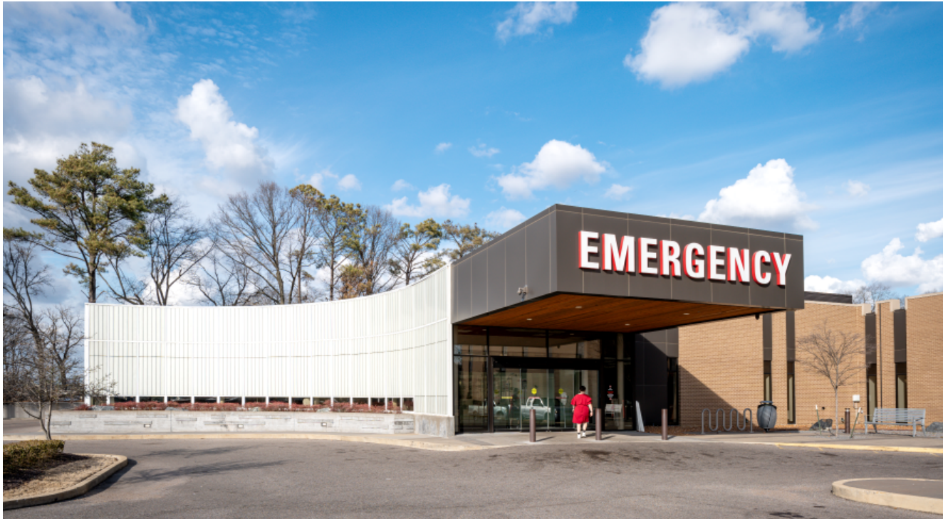
Figure 6a. The translucent wall at this hospital maximizes daylight while moderating heat gain.
