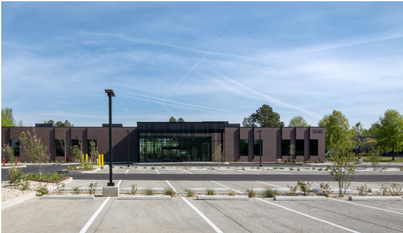
Figure 4a. The water-wise landscaping subtly softens the parking lot, creating bioswales that, in tandem with porous paving, capture stormwater runoff.
