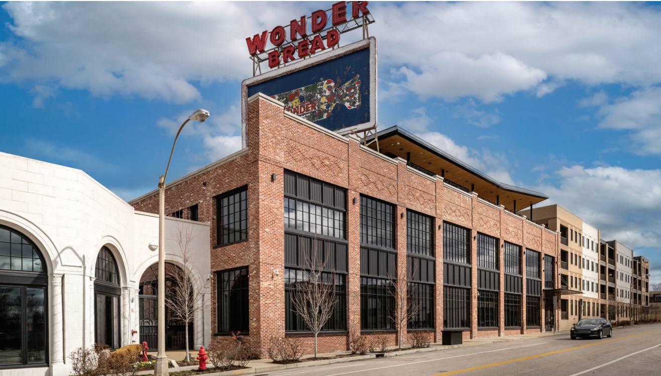
Figure 9a. This renovated facade was repaired with bricks salvaged from buildings in the surrounding area.
