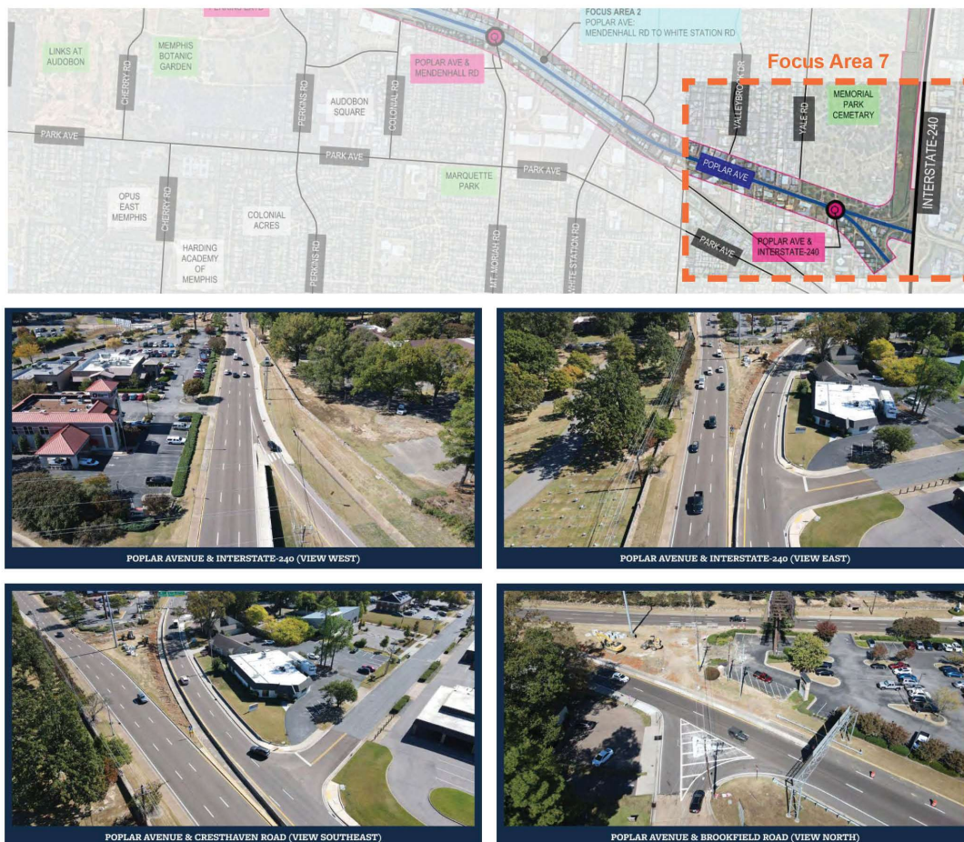
Figure 39: Poplar Avenue at I-240 Existing Conditions
