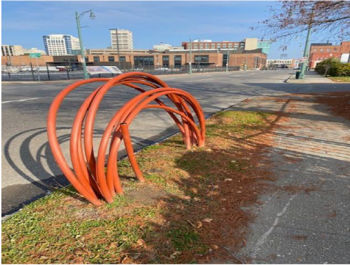
Figure 6.3: Examples of Unacceptable Fiber Route Termination
