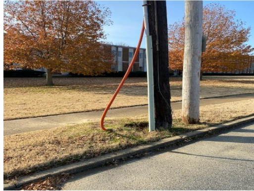
Figure 6.3: Examples of Unacceptable Fiber Route Termination
