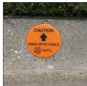
Figure 6.3: Acceptable Fiber Route Marker
