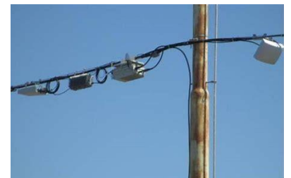
Figure 2.5: Acceptable Strand Mount
