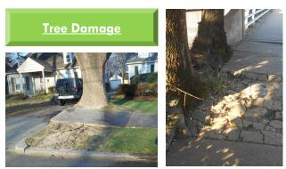
**Solution:** Replace Damaged Sidewalk Panels, Mitigation of Tree Roots or Tree Removal May Be Required
