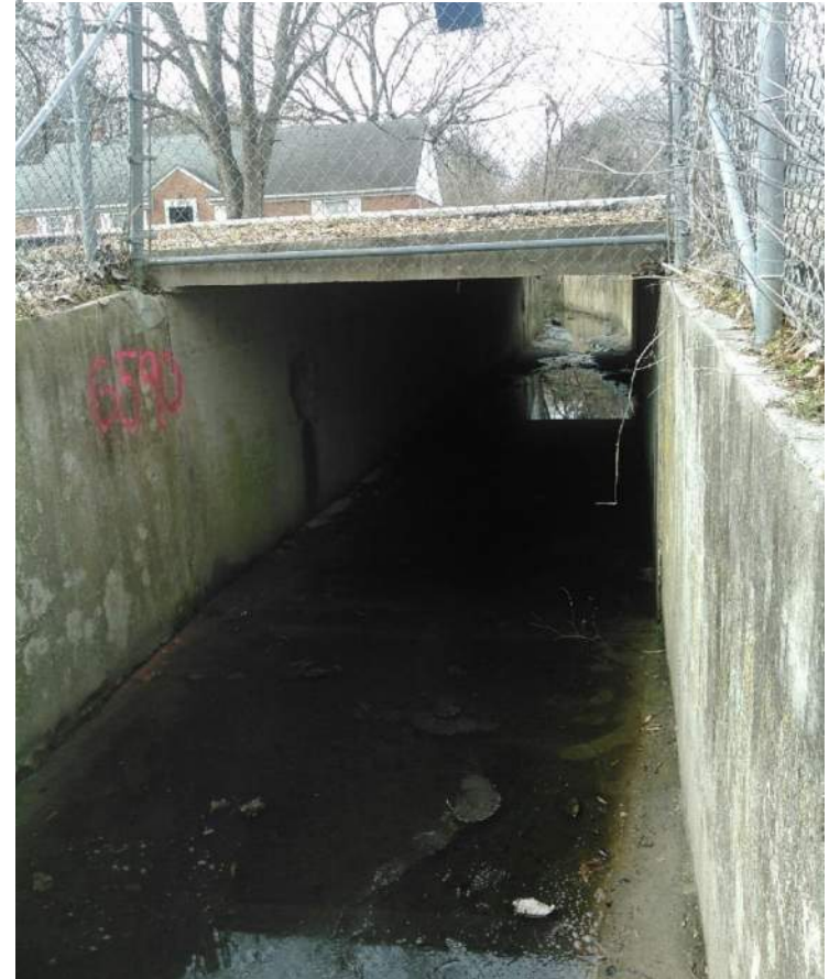
Crossing under W Rosita Circle south of E Brooks Rd.
